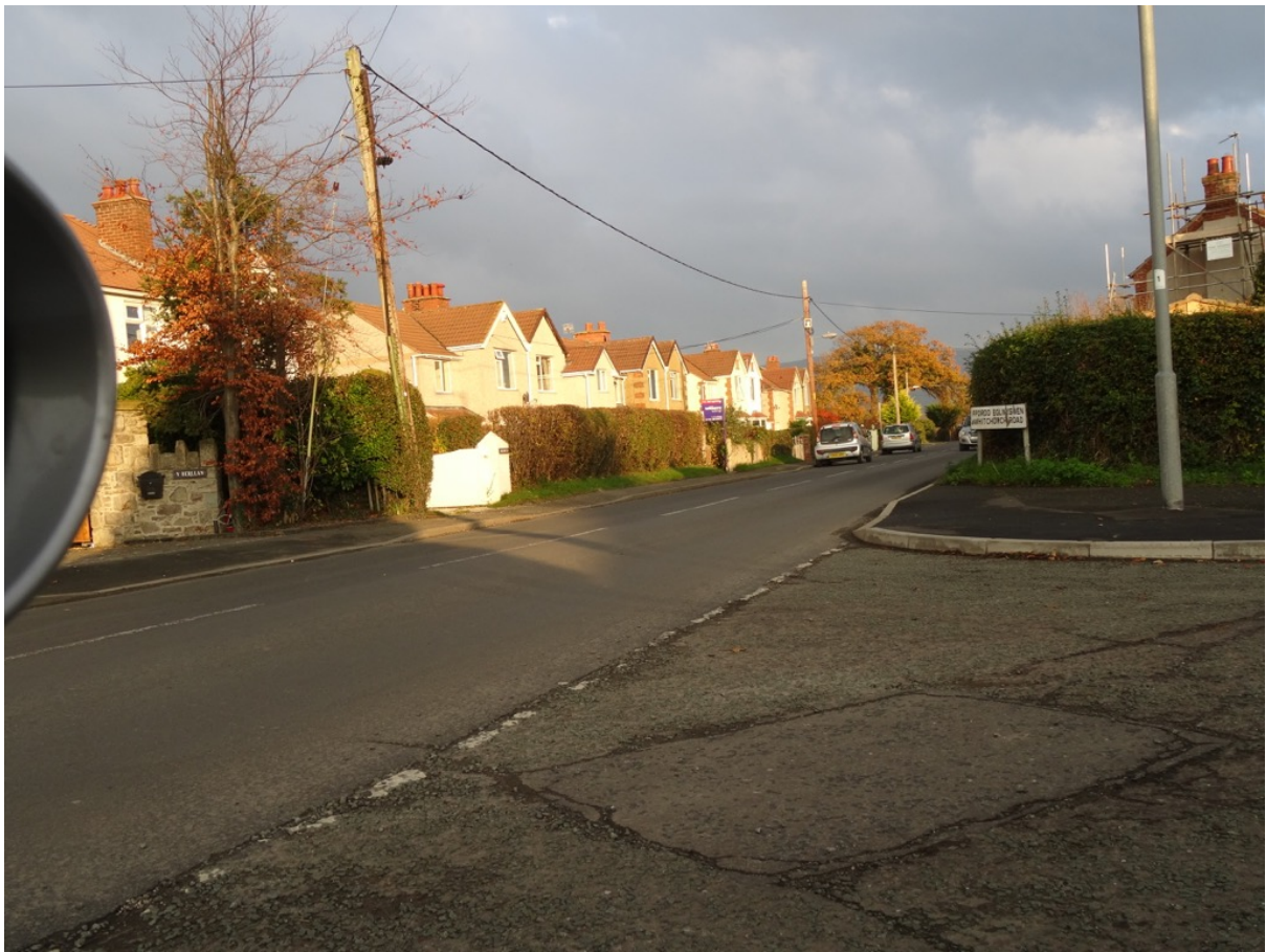
Photo 7 – Junction from Old Ruthin Road to Whitchurch Road
